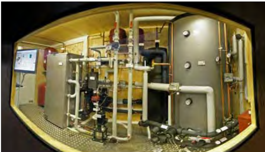
◀ Figure 3. Indoor components of the solar cooling installation at the office building of the Company SOLID in Graz, Austria (17.5 kW Yazaki chiller WFC 5). (Source: SOLID)
