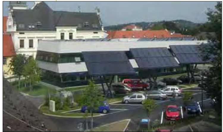
▲ Figure 2. Solar heating and cooling installation at the Town Hall Gleisdorf, Austria (304 m 2 flat plate collectors connected to 35 kW Yazaki chiller WFC 10 and a desiccant evaporative cooling system). (Source: AEE INTEC)
