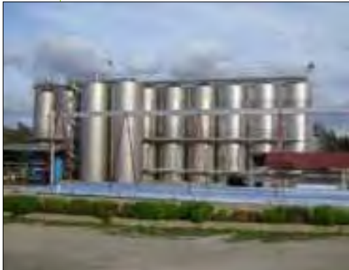
The solar cooling system installed at this Tunisian winery was monitored by Task 38 experts and received the Energy Globe Award Tunisia 2009.
