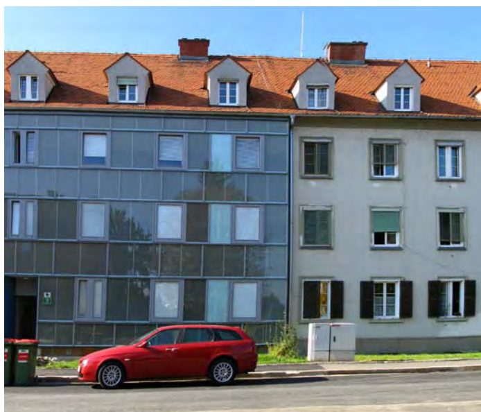
Figure 3. Refurbished row house at Dieselweg in Graz (left) and original situation (right).
