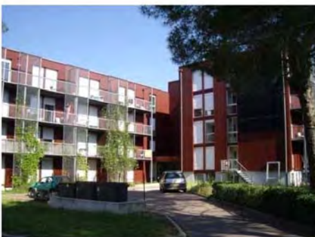
Figure 1: South view of the building after retrofitting
