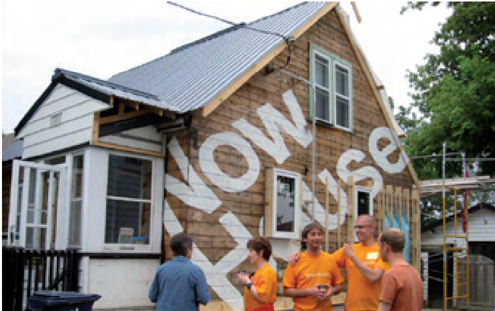
The first Now House Project in mid-construction, Topham Park, Toronto 2007-2008
