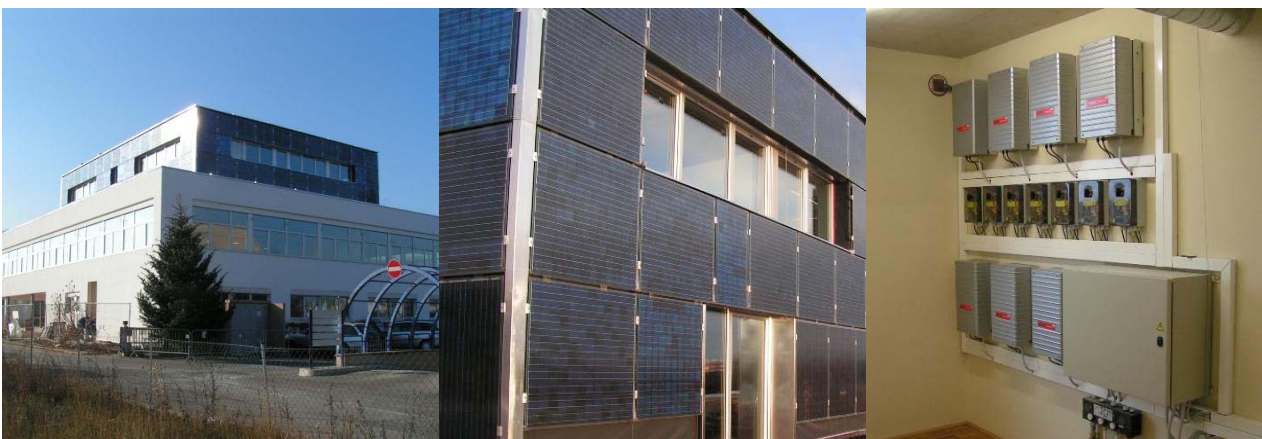
Figure 5 Photovoltaic cladding system and building services control room with grid-tied supply switching system, designed and installed by ATB Becker, Absam, Austria.
