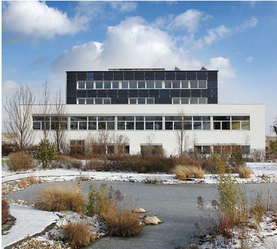
Figure 1 East façade of SOL4, January 2005 (SOL4 2005, photo courtesy of Thomas Kirschner).
