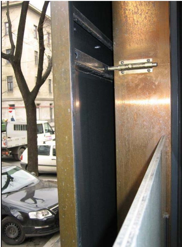
Abb. 20: Detail Fenster [Quelle: Boku, Wien]
