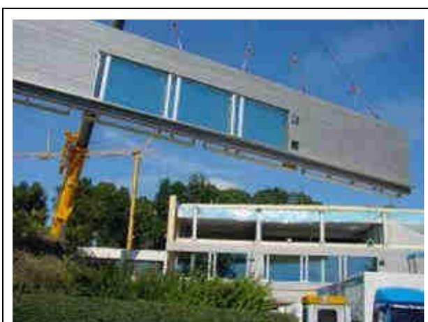
*Figure 1 Integrated wooden frame windows and solar shading in a big prefabricated timber module for renovation of a school façade (Source: PAUAT Architekten)*
