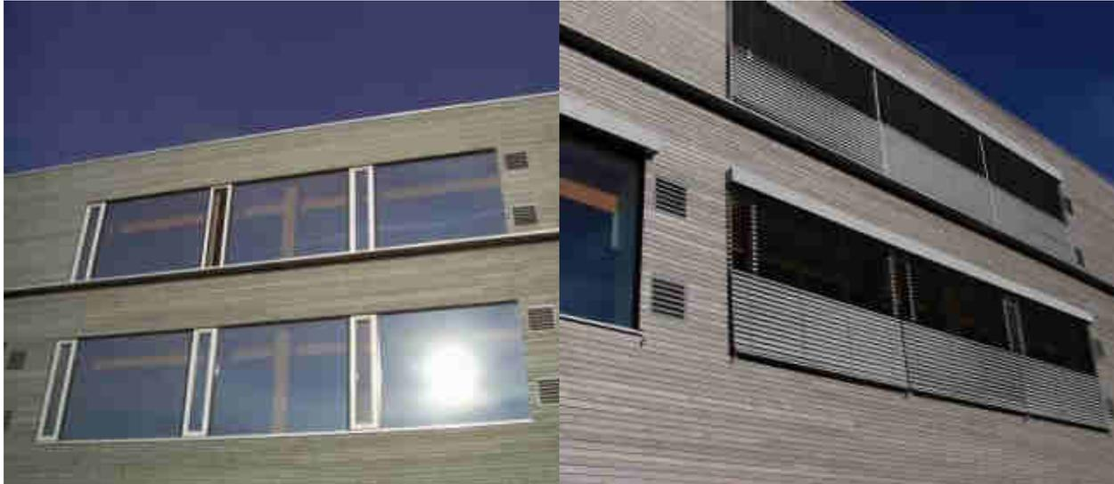
*Figure 25 Missing external shading in the first year (left picture) caused overheating in the classrooms of the New Secondary School Schwanenstadt. As reaction to this an external shading system was installed in the second year (right picture).*
