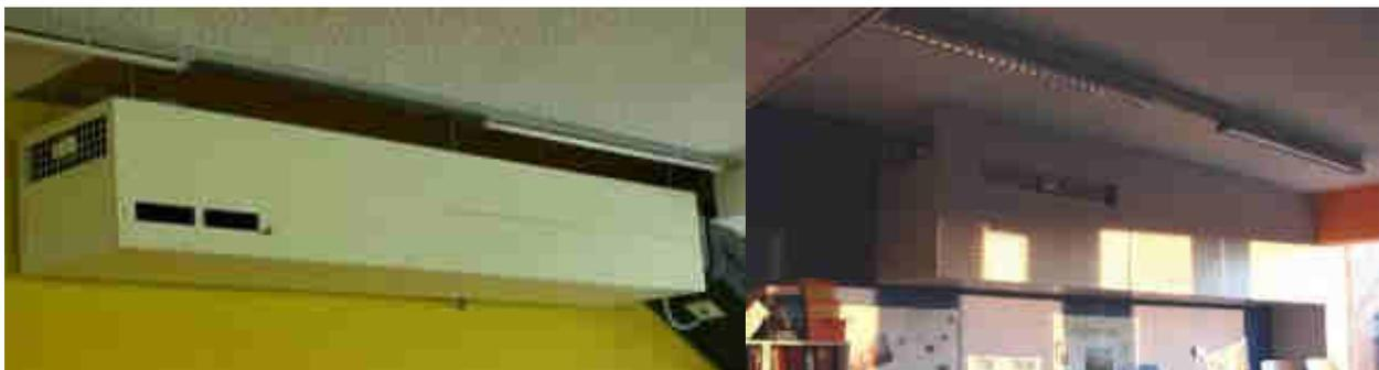
*Figure 26 Missing housing of decentralised ventilation units caused sound problems in the first operated model classroom (see left picture). The housing was installed regularly later (right picture) to improve the situation in the classrooms.*
