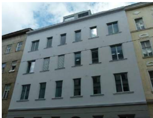
Object Eberlgasse (Eberl Alley) - First modernization of a historic building to passive house standard - water/water heat pump - air ventilation system
