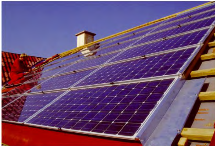
Laminate modules roof with Solrif mounting
