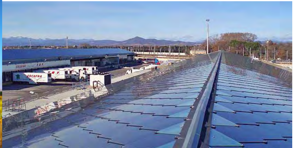
Marché Saint Charles (Perpignan, Aude) – 8.8 MWp BIPV installation
