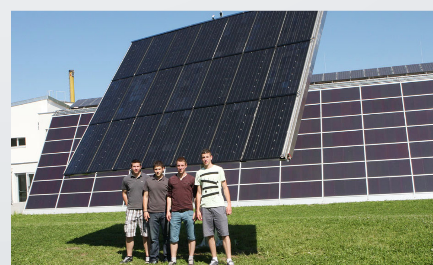
Fig. 6: Dual-axis tracking system (Source: FH FJ Wieselburg)
