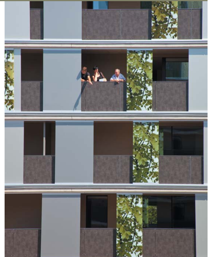
Fassade B2 | Facade B2
