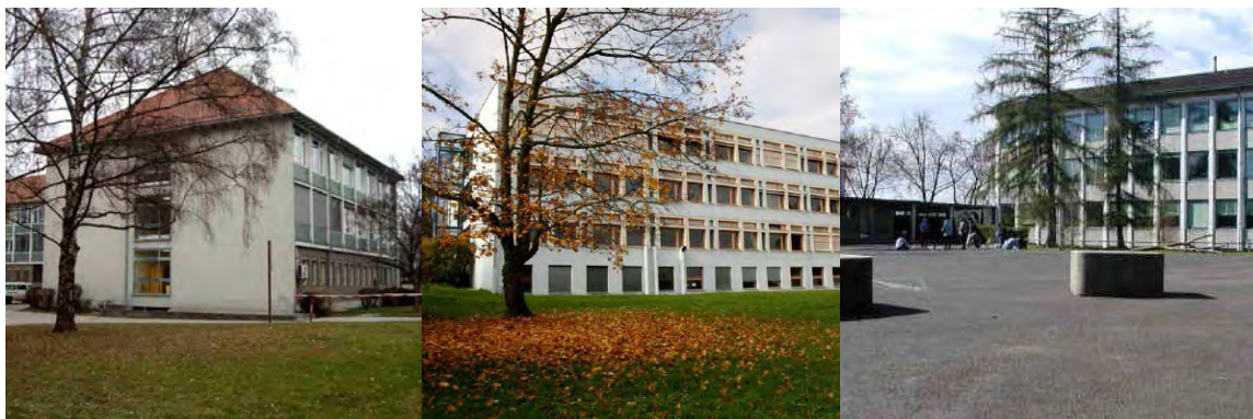
Figure 6 Skeleton façades on the example of the case study buildings A02 (left - AEE INTEC), CH01 (middle - CCTP) und CH08 (right - CCTP)
