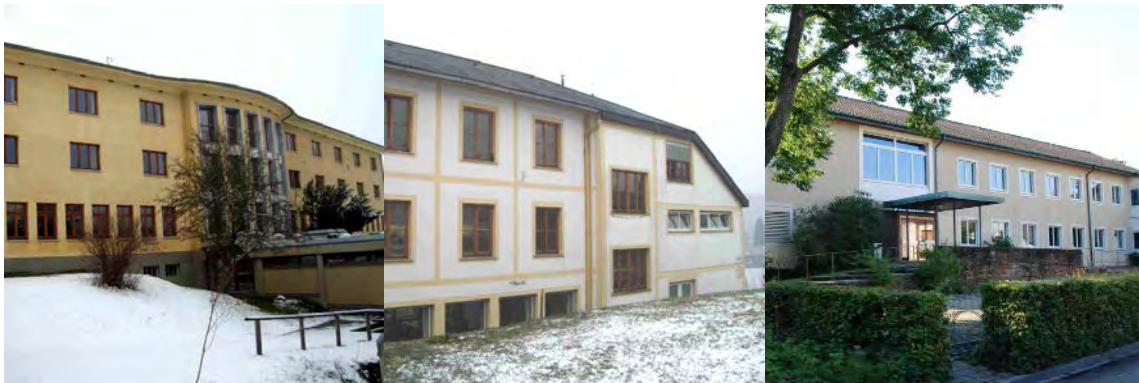
Figure 4 Punctuated façades on the example of the case study buildings A03 (left - AEE INTEC), A05 (middle - AEE INTEC) and CH04 (right - CCTP)
