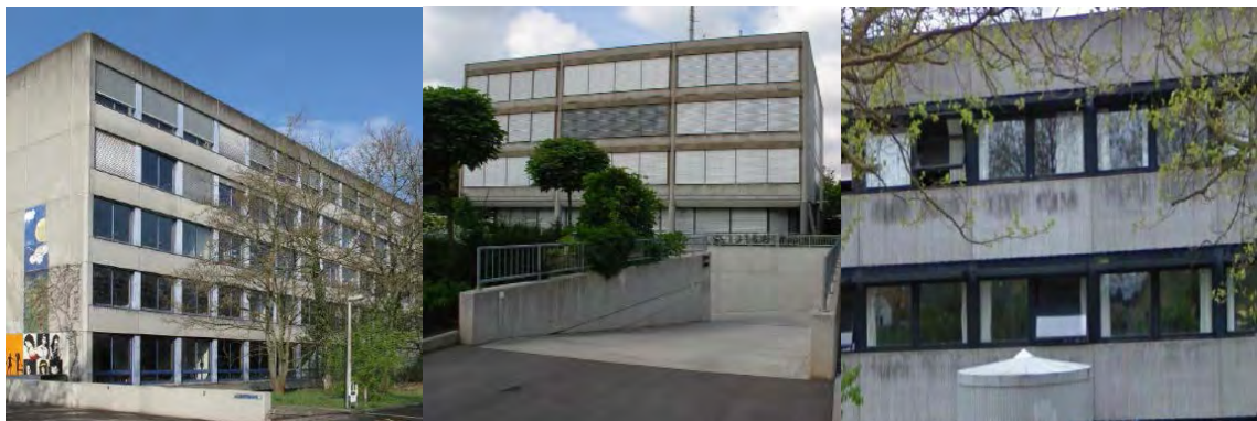
Figure 5 Element based façades on the example of the case study buildings CH05 (left - CCTP), CH07 (middle - CCTP) und DK02 (right - DTU)
