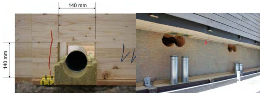
Figure 38 left: Detail of a ventilation duct during production of the facade modules in the factory right: Joining of two modules during assembly with ventilation ducts at the building site
