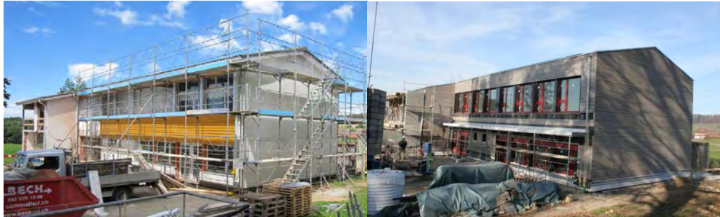
Figure 36 View of the Krumbach building at the begin of renewal (left) and before finishing (right)
