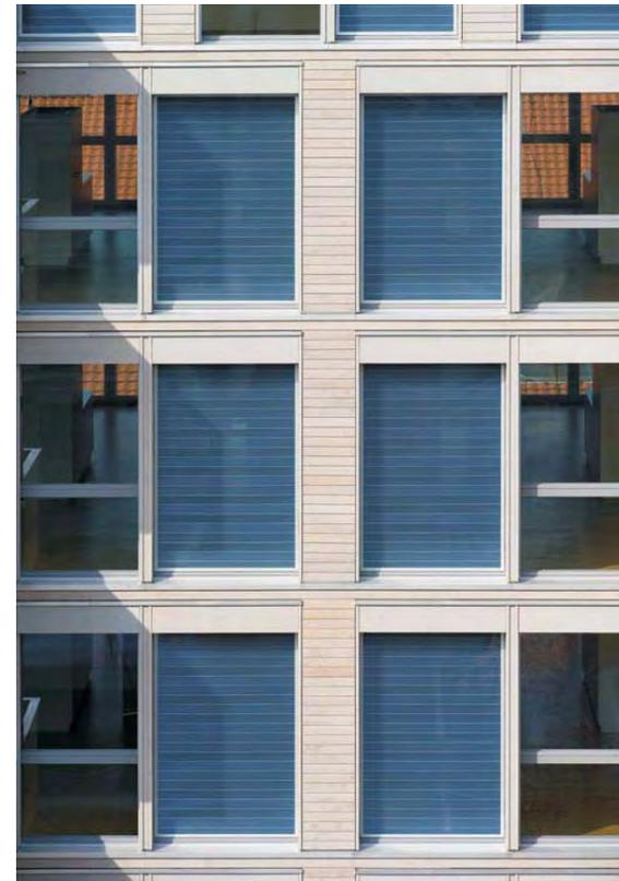
These multilayer solar crystals (GLASSXcrystal) have the effect of heating during wintertime and cooling in summer.
