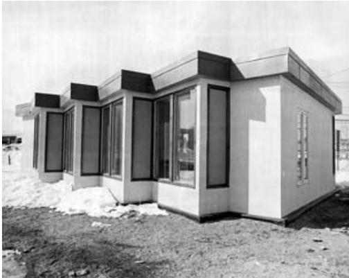
**Solar V** was erected in 1978 on the MIT campus and used as an experimental studio/classroom by the Department of Architecture. Unlike the first four solar houses, Solar V did not require mechanical equipment such as solar collectors, pumps or fans: all elements of solar heating were incorporated into the building materials.
