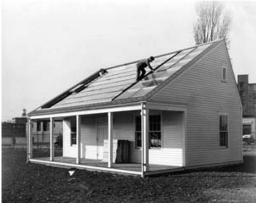
**Solar I**, completed in 1939, was the first house in America to be heated by the sun's energy. A single story house-like structure on the MIT campus, Solar One used solar radiation as a heat source for the winter, but projects were also conducted on summer air conditioning and power generation.
