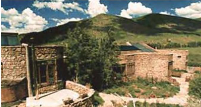
Amory Lovins, a well known author of books for alternative energy use, built in Old Snowmass, Colorado (2164 m high) a super insulated house with super windows (heavy-gas-filled Heat Mirror® windows) and passive solar gains. The active solar panels drive an under-floor radiant heating system and the domestic hot water system. Tropical plants grow in the winter garden and the oven is used very rarely.
