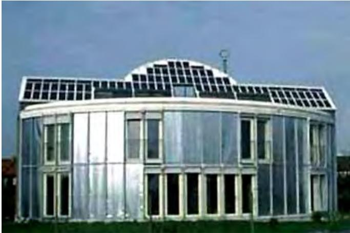
The “Energy-Autarc-Solar-House” (ISE, Freiburg 1991/92, by Wilhelm Stahl) was built at the same time as the Passive House Darmstadt-Kranichstein. It is very near to the Passive House Standard. The very complicated hydrogen-storage technology is no longer used. The passive technology and the heat recovery ventilation are working well and today it is used as a Passive House.
