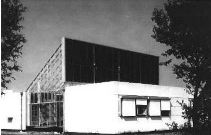
The Dansk "DTH-Zero-Energy-House," built in 1973 in Lyngby by Vagn Korsgaard and Torben v. Esbensen from the Thermal Insulation Laboratory, was a Passive House designed according to simulation calculations.
