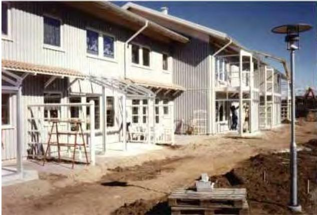
In 1985 the Swedish pioneer and architect Hans Eek built super-low-energy-houses with 30 kWh/(m<sup>2</sup>a) heating demand in Ingolstadt-Halmstadt.
