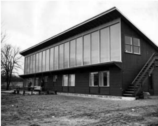
The **Solar VI** house is the Dover Sun House. The heating storage device was Glauber salts (sodium sulphate decahydrate). After 3 years the system failed.
