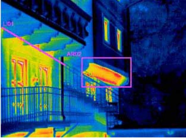
A thermal image of a building corner at night. The image shows a balcony with a metal railing. The walls are mostly blue, but there are red and yellow areas at the base of the walls and on the balcony floor, indicating heat loss. A pink box highlights a specific area on the balcony. Labels 'L101' and 'AR02' are visible in the image.                                         |
