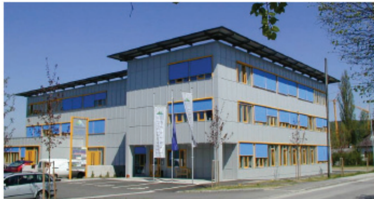
Technologiezentrum Salzammergut in Attnang-Puchheim
