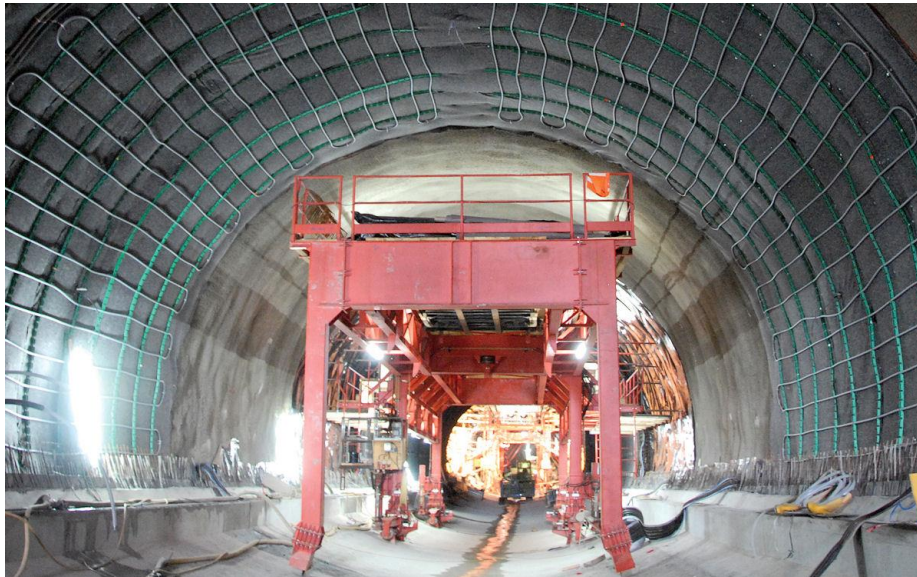
Figure 25: installation of absorber pipes in a tunnel [16].
