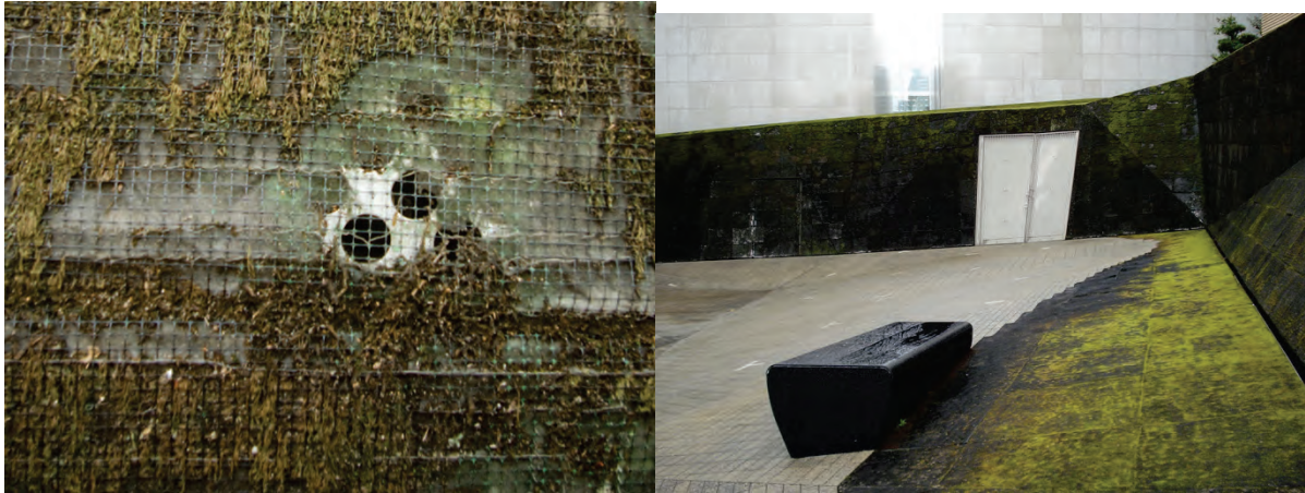
Abbildung 50 (links): Prada-Store Tokyo, Detail Moospanel Bildquelle: https://www.flickr.com/photos/jrosenk/3103127649/in/photostream/(Jessica Rosenkrantz) ; Abbildung 51 (rechts): Prada-Store Tokyo, Mooswand Bildquelle: https://www.flickr.com/photos/atelier_flir/4459686155/ (Timothy Brown)
