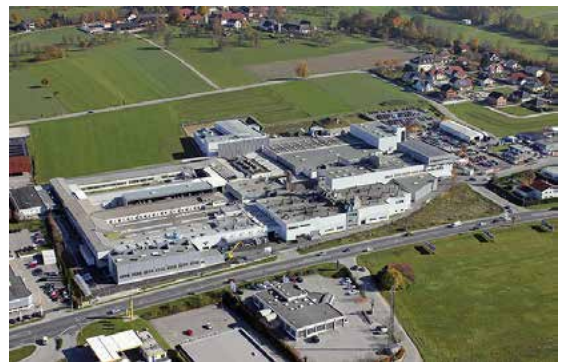
Plant 1 – Kirchdorf/Krems, Photo: TCG UNITECH GmbH
