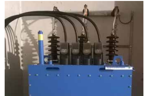
Residential PV storage system and onload tap changer Köstendorf, both photos: Salzburg Netz GmbH
