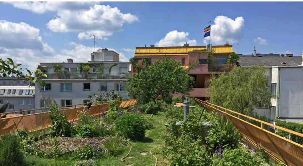
Greenery on a roof through urban gardening, Sargfabrik, Vienna; Photo: GRÜNSTATTGRAU
