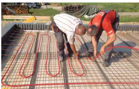
Installing a thermally activated building system in the top level of a ceiling, Photo: Aichinger Hoch- und Tiefbau GmbH
