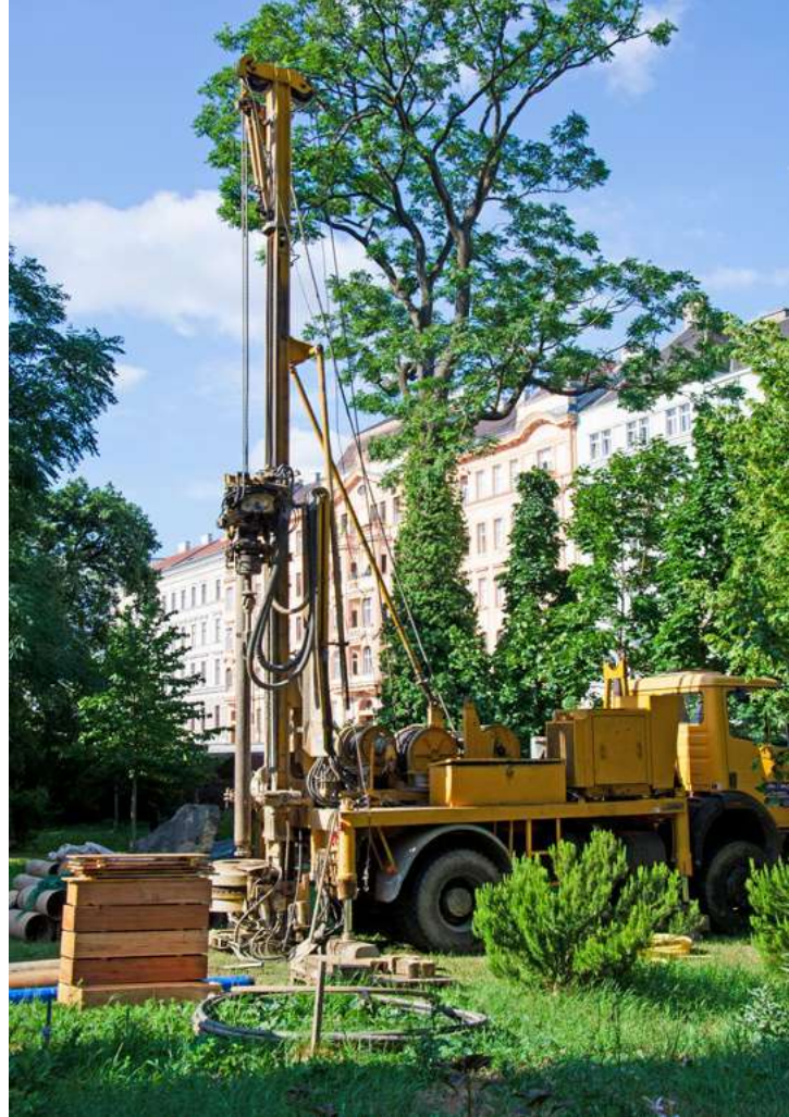
Drilling the test geothermal probe, photo: Heat Harvest consortium
