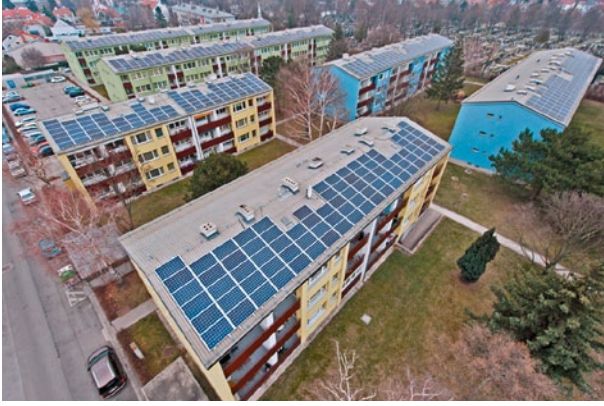
The city as a power station - PV facility owned by Wien Süd in Vienna's 23rd district, Photo: Wien Süd
