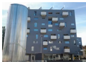
Stadtwerk Lehen - Solar storage tank, Photo: SIR
