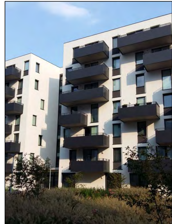
Fig.: Exterior view of building 2 source: Peter Holzer
