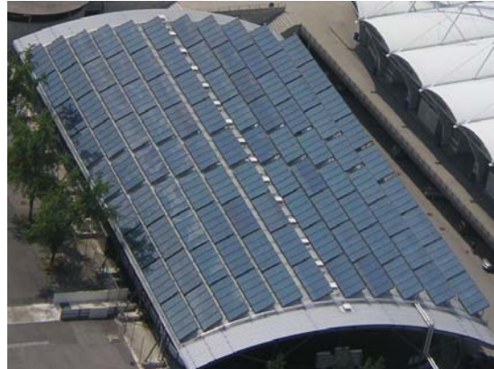
Fig. 3 Solar thermal plant, football stadium "UPC-Arena" in Graz, Austria (Source: SOLID, Austria)
