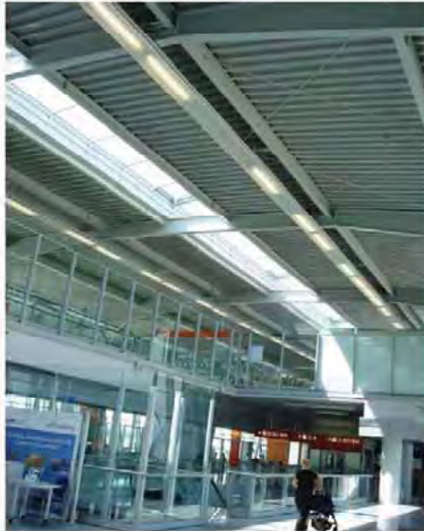
Lack of control
