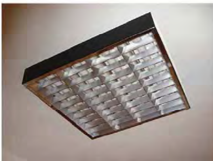
Antiquated (> 20 years old) T12 – Louver - Luminaire
