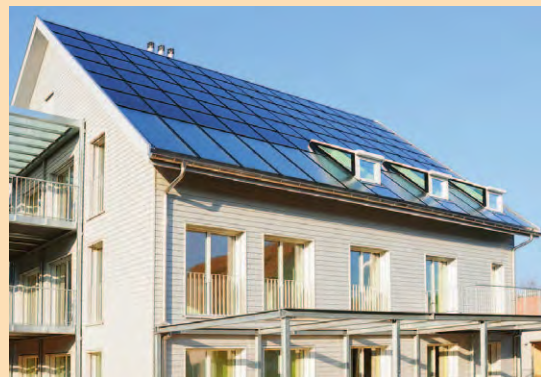
PV and solar thermal combined on a Swiss house, courtesy SOLTOP AG
