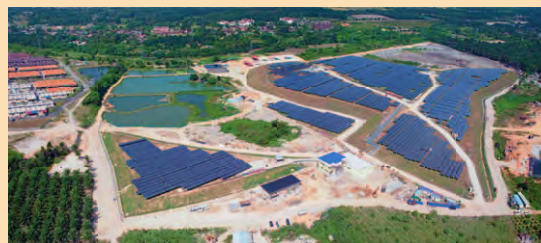
8 MW PV on landfill, Pajam, Malaysia
