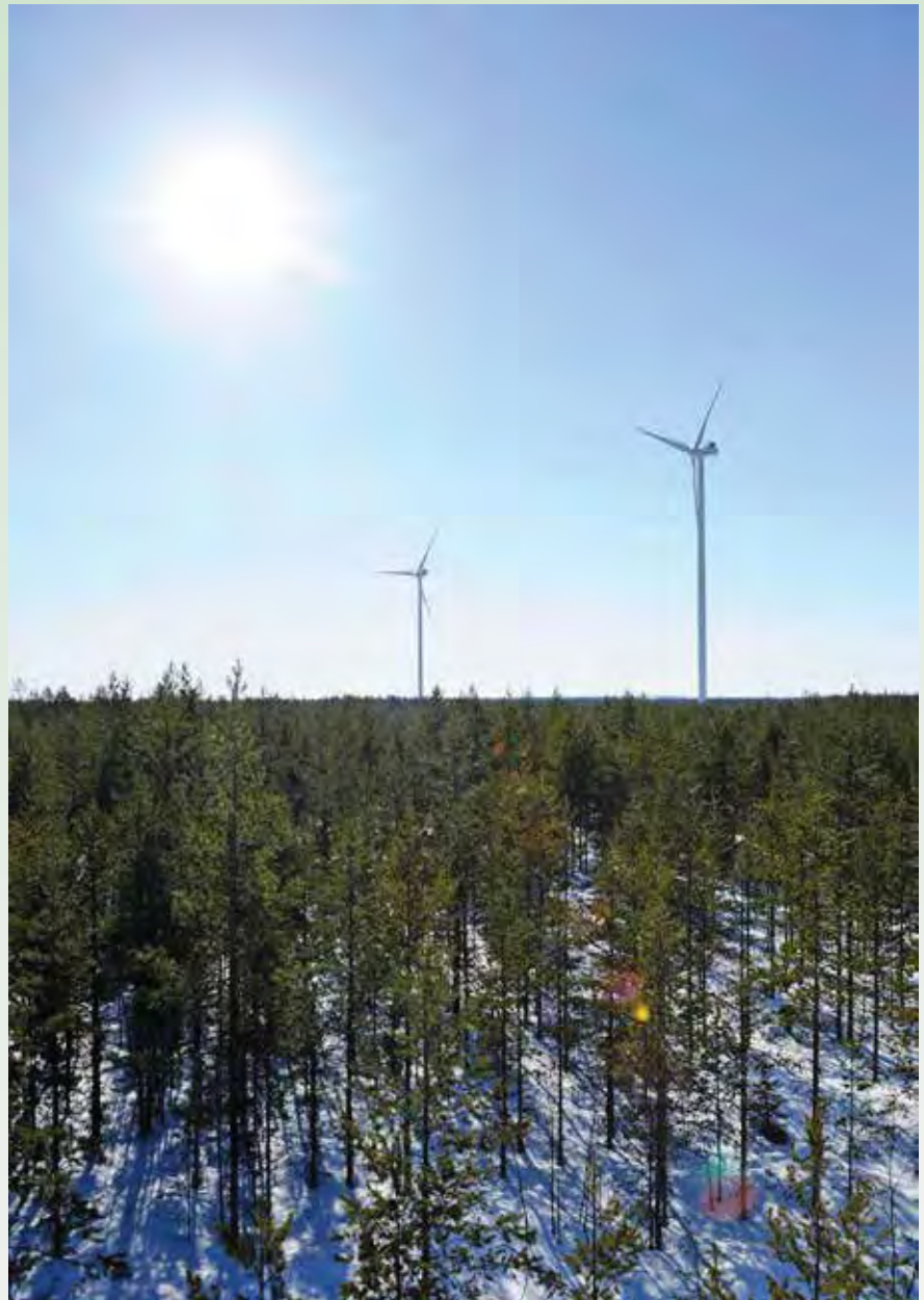
Figure 4. Olhava wind power plant. (Source: Tuuliwatti)
