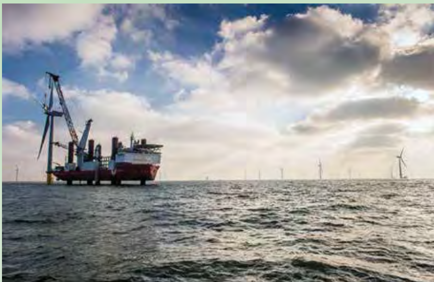
Figure 2. Installation of final turbine in first 630-MW phase of the London Array Offshore Wind Farm. Courtesy: London Array
