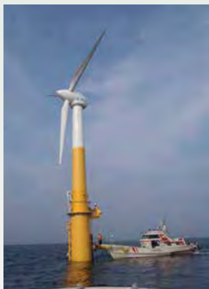
Figure 3. A small-scale floating offshore wind turbine (SUBARU 22/100 100-kW) installed 1 km offshore in Nagasaki Prefecture in the MOE Floating Offshore Wind Turbine Project
