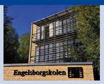
Fig. 1 - 6 kWp mono crystalline PV integrated as shading system in the facade of the school Engelsborgskolen in Copenhagen, developed by Gaia Solar.
