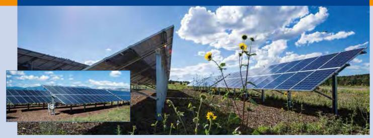
Fig. 3 - 67 kW (STC rating) photovoltaic array at the Mesa Verde Visitor and Research Center in Montezuma County, Colorado. The array consists of 286 Schott Poly 235 watt solar modules (13,8 % efficiency) wired in 22 series strings of 13 modules per string. Coupled with a micro-hydro system and solar water heating, the on-site renewable energy systems are capable of providing 95 % of the building energy requirements (Photo: Dennis Schroeder / NREL).
