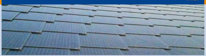
Fig. 3 - 12 kWp PV plant at Borgoricco (PD), using SAINT-GOBAIN SOLAR rigid modules on tiles (SI crystalline cells) (Photo: GSE, Gestore del Sistema Elettrico).
