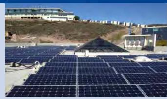
Fig. 2 - 75 kWp Grid Connected PV System at CICESE Ensenada Baja California, Mexico (Photo: Solartec).
