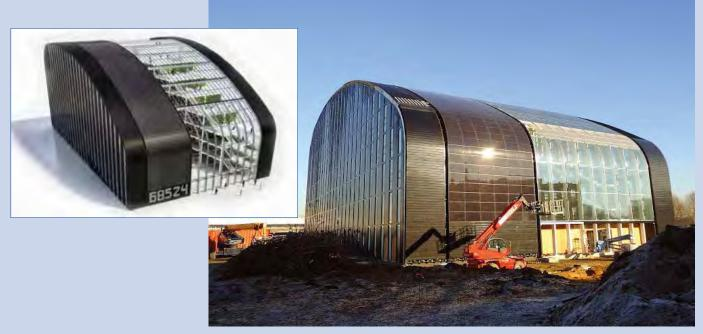
Fig. 1a & Fig. 1b - Bruxelles Environnement. The new Brussels Environment and Energy Administration Headquarters will be the largest passive office building in Europe and will include 700 m<sup>2</sup> of BIPV ISSOL modules (Photos: Copyright CEPEZED, ISSOL for Fig. 1a and ISSOL for Fig. 1b).
