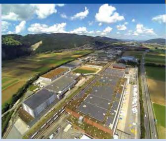
Fig. 4 – Migros Logistics Centre, Neuendorf, Switzerland. 5,2 MW on-roof PV system (Photo: Tritec AG).
