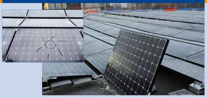
Fig. 4 - PV installation at Powerhouse Kjørbo, delivered by Direct Energy. The system has a capacity of 310 kWp (See also www.powerhouse.no).
