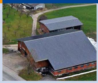
Fig. 2 - Farmhouse in Sempach , Switzerland. 171 kW roof-integrated PV system (Photo: Schürch-Eqli AG).
