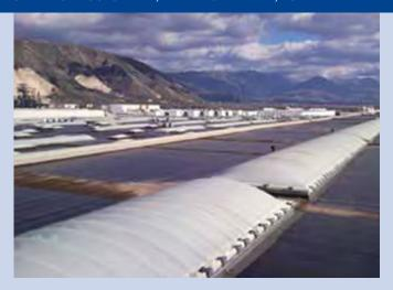
Fig. 1 – 1 544 kWp PV plant at NoIa (NA), using General Solar Flexible Modules (thin film on flexible support) (Photo: GSE, Gestore del Sistema Elettrico).
