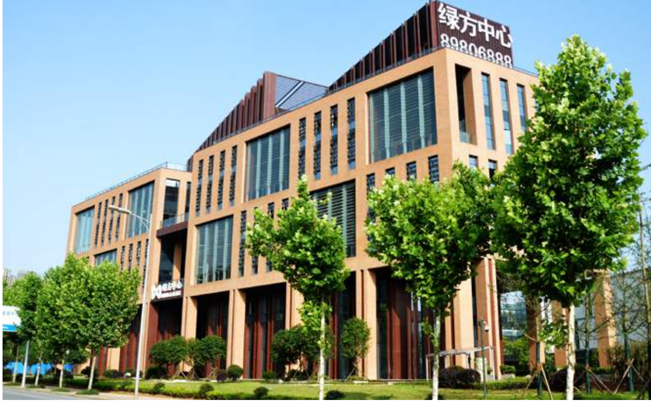
Fangxing Green Building Exhibition Center, Meixi Lake, Changsha, P.R. China. The building uses ventilative cooling through automatic window opening in mid season conditions. Source: Liang Tang
