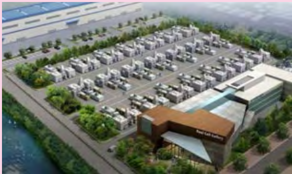
Figure 8: Artists impression of the completed Hwasung 58MW site, currently under construction.
