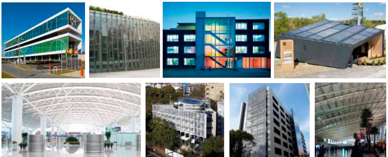
Case study buildings of high temperature cooling and low temperature heating systems. Clockwise from top left: Bayer Diegem in Belgium, EWHA Women's University Campus Center in South Korea, Energy-plus house in Denmark, Danish Solar Decathlon House in Denmark, Xi'an airport Terminal 2 in P.R. China, a campus building of Nagoya University in Japan, Museum of Earthquake Reduction in Japan, Xi'an airport Terminal 3 in P.R. China.
