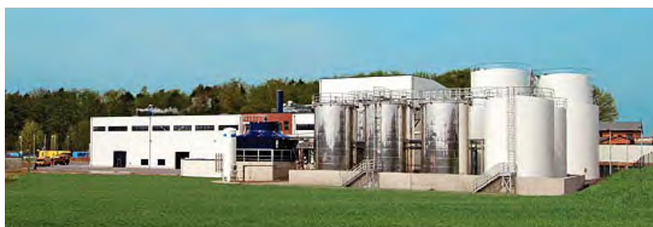
Figure 9. The biodiesel plant Sternberg/Germany.
