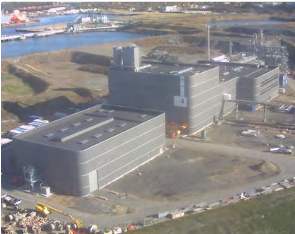
Figure 14. The bioethanol plant in Kalundborg/Denmark.
