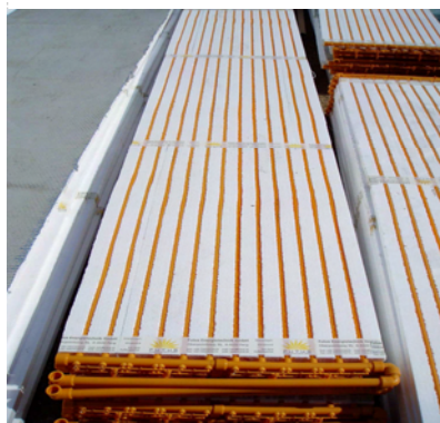
Figure 13: Heating pipes are inserted in XPS boards, which are mounted onto the existing wall.
