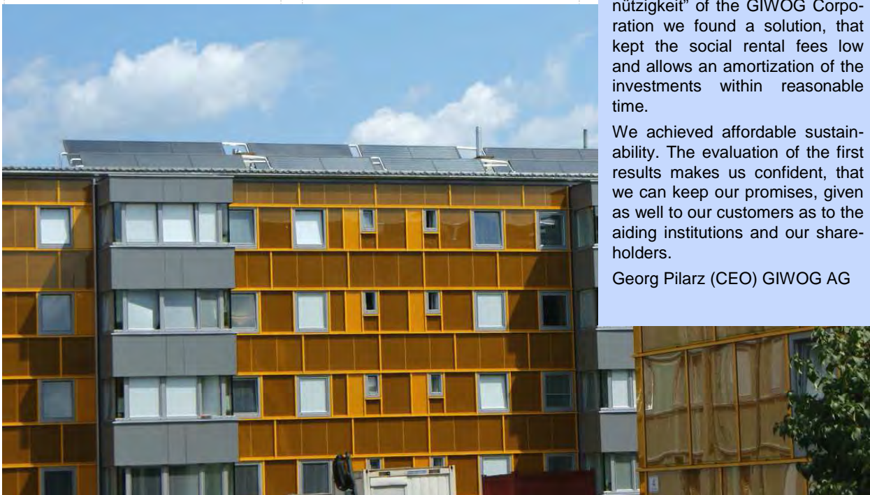
Figure 21: View on the finished façade – showing the new façade structure with integrated windows and balconies, and the solar thermal collectors on the flat roof
