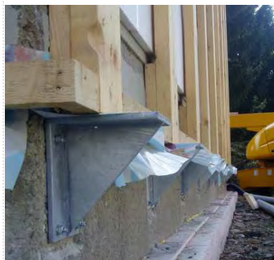
Figure 17: Steel-bearing angles on the plinth.
