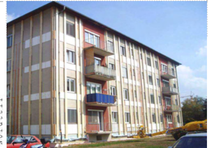
Figure 12: Heat dissipation – XPS-boards installed on existing façade.
