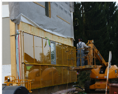
Figure 16: Assembly of the lowest module
