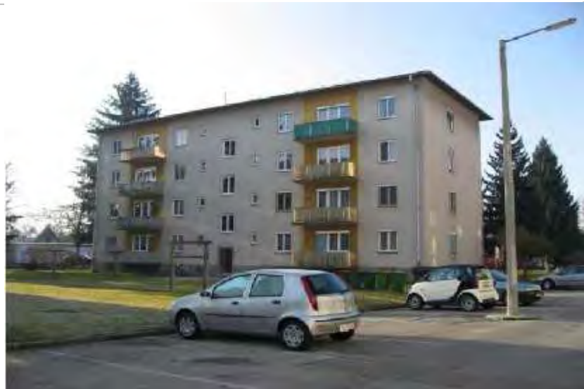
Figure 1: View of building [source: GIWOG]
