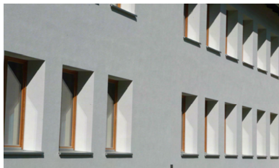
Picture 7-4: Windows mounted centered within reveal (Source: Obereder H., A+ ZT GmbH)
