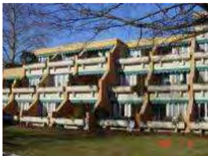
Picture 2-4: Building stock – plate construction type (Source: Ziv. Ing. Büro Boder)
