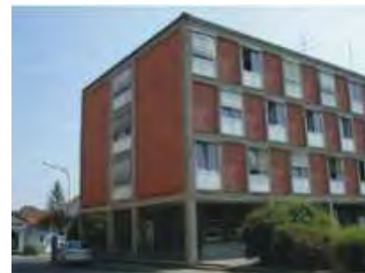
Picture 2-5: Building stock – skeleton construction (Source: LIG Steiermark)
