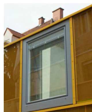
Picture 7-7: Blinds mounted "intermediate" (in-between the glass-panels) – to be used for plane façades. (Source: AEE INTEC)
