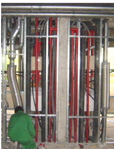
Picture 9-1: Installation module inside the building (Source: Ziv.Ing. Büro Boder)
