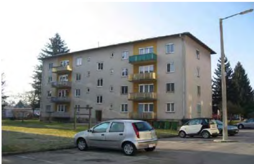
Figure 1: View of building (source: GIWOG)
