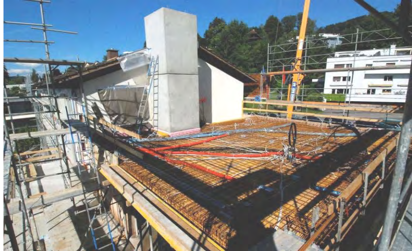
Figure 12: Construction of building annex with two additional apartments
