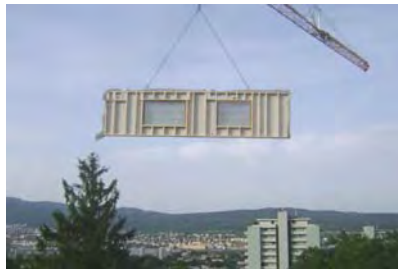
Figure 20: Mounting of 3 m by 10 m façade elements
