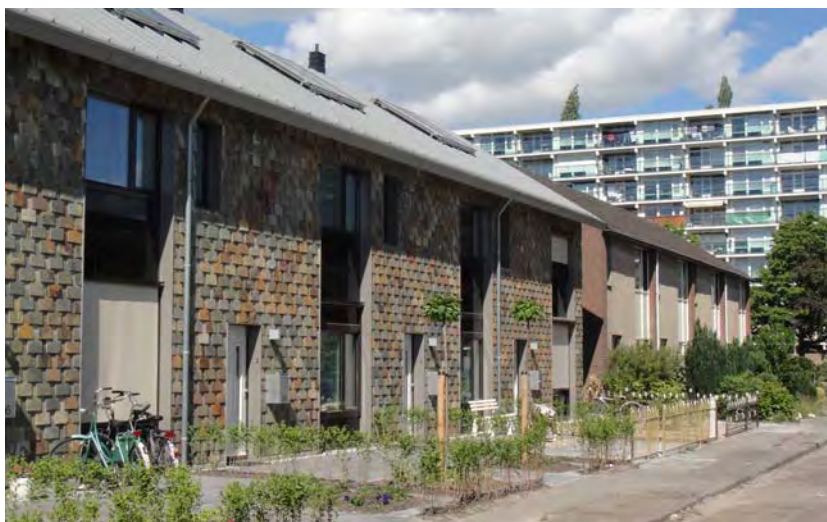
Figure 13: Impression of renovated and unrenovated houses
