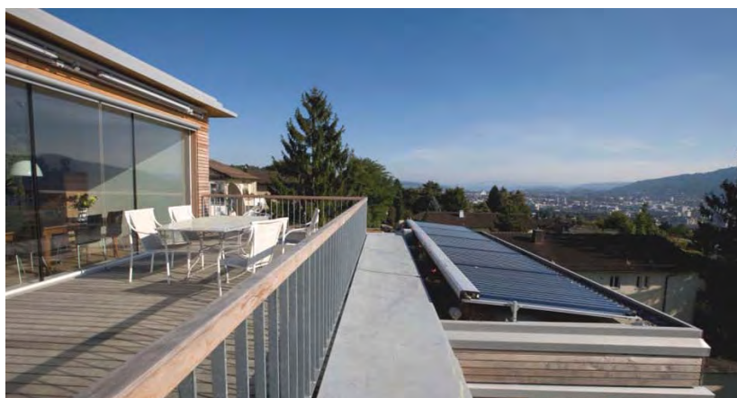
Figure 29: View from new penthouse terrace over Zurich, with 12.5 m 2 vacuum solar collectors on the balcony roof
