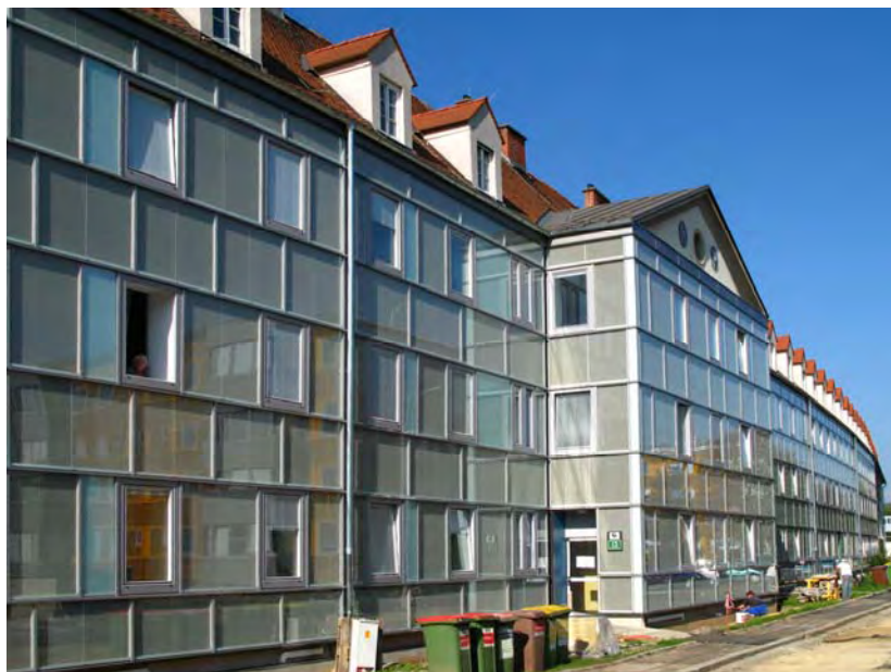
Figure 4: Dieselweg 3 and 19 – covered with new façade modules
