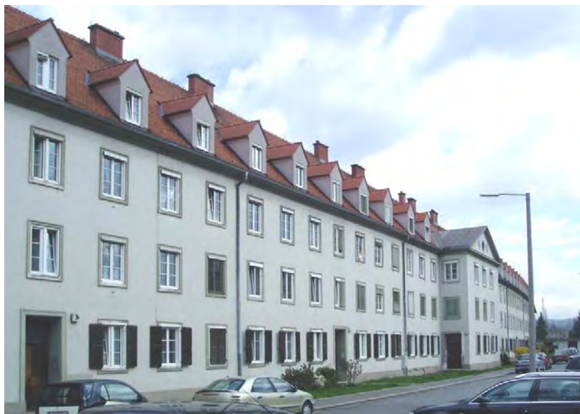
Figure 1: View of "Dieselweg 3-19" before renovation
