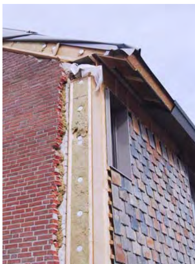
Figure 4: Section of renovated building
