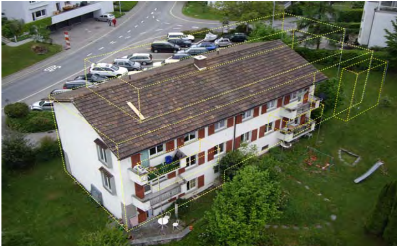
Figure 4: View of old building and project
