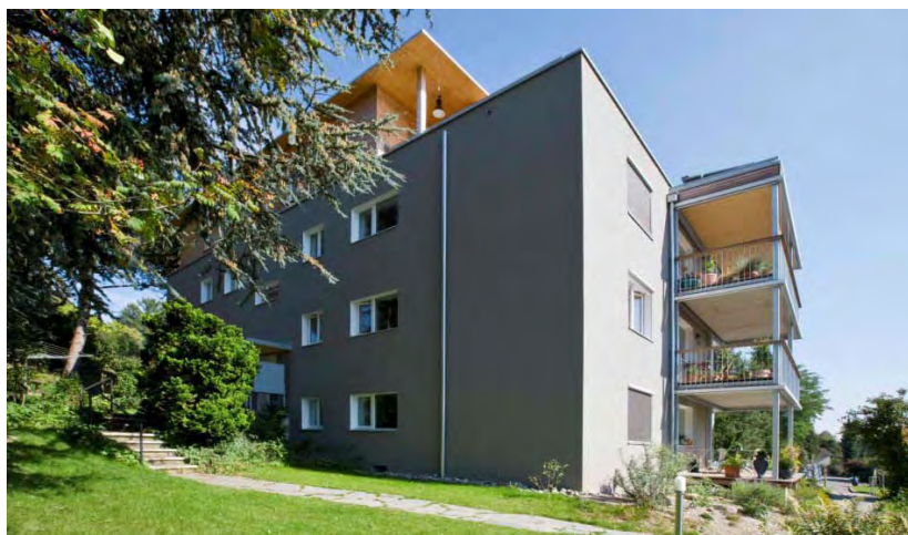
Figure 28: Renovated building from west side
