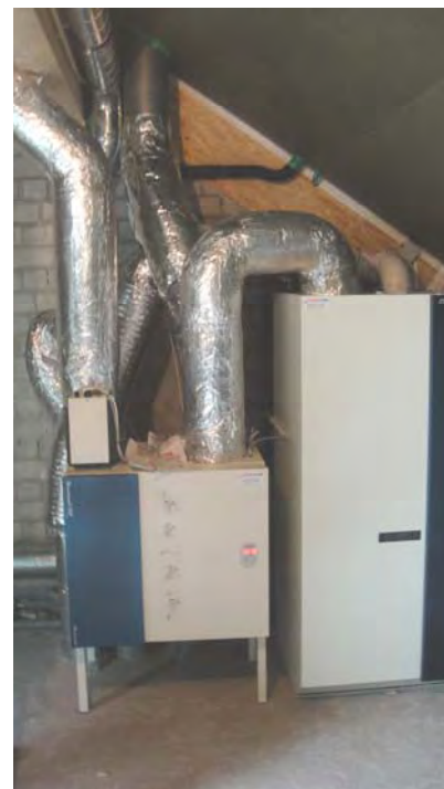
Figure 7: Combined heating, ventilation and hot water system
