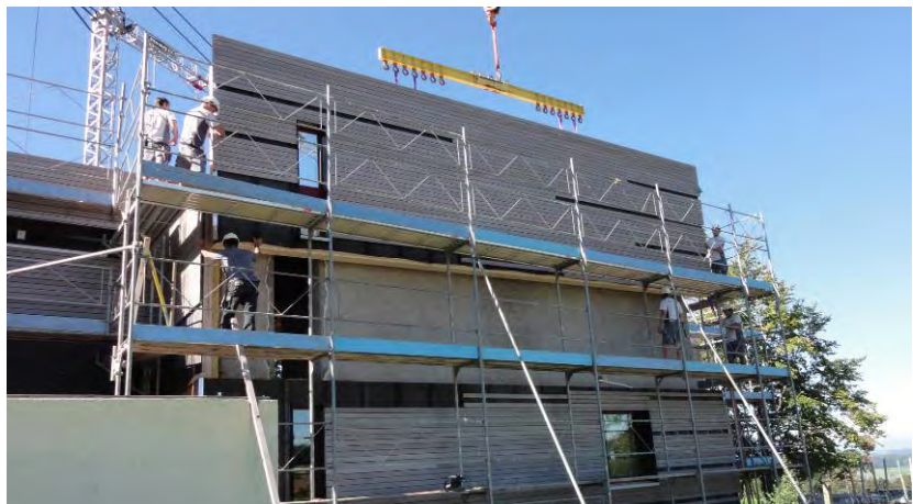
Figure 21: Mounting of the second module row
