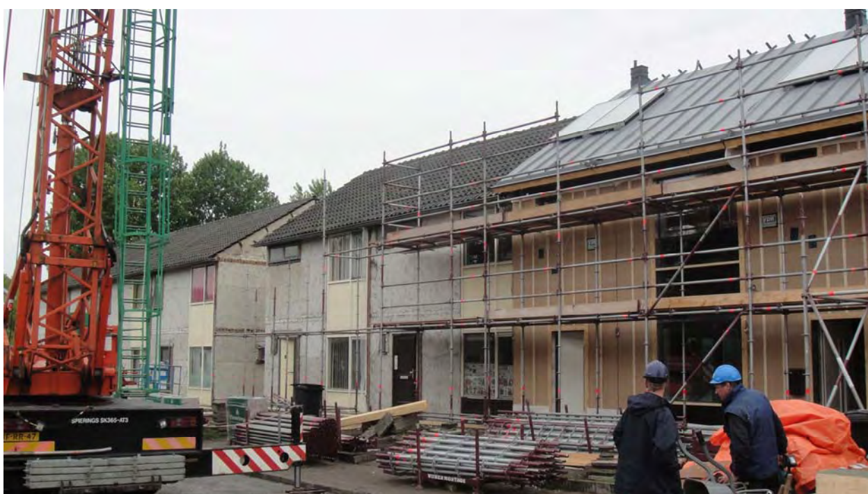
Figure 11: Renovation in progress: one house per day
