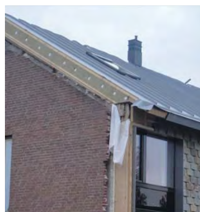
Figure 10: Prefab elements mounted on site
