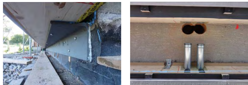
Figure 19-20: Horizontal mounting angle and a modules just before its final position
