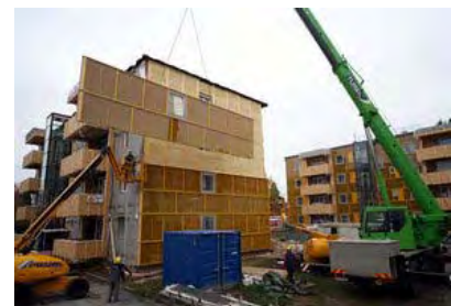
Figure 20: Mounting of 3 rd module
