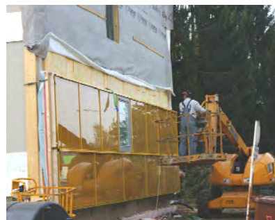
Figure 19: Assembly of lowest module
