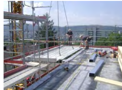
Figure 24: Mounting of the living room extension
