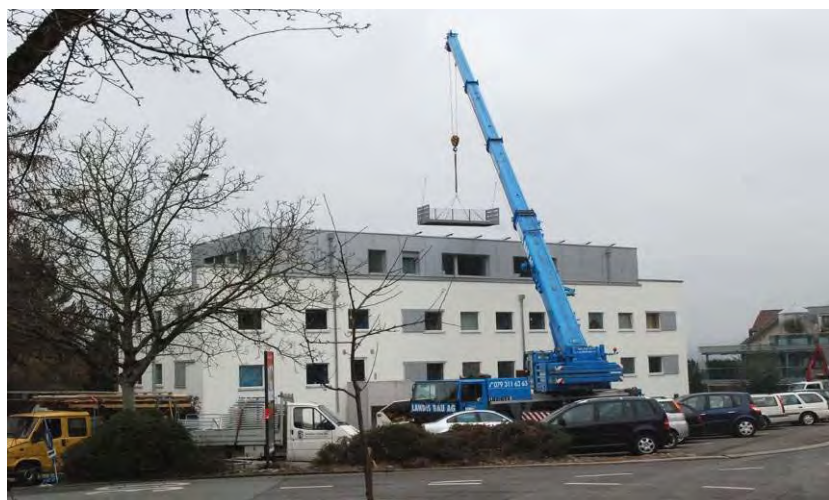
Figure 15: Mounting of pre-fabricated balconies
