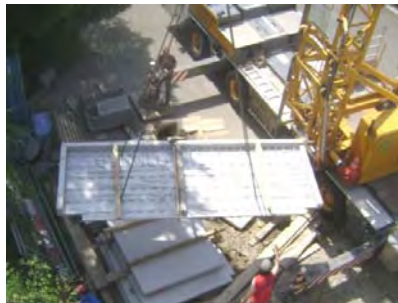
Figure 23: Prefabricated roof element for the living room extension
