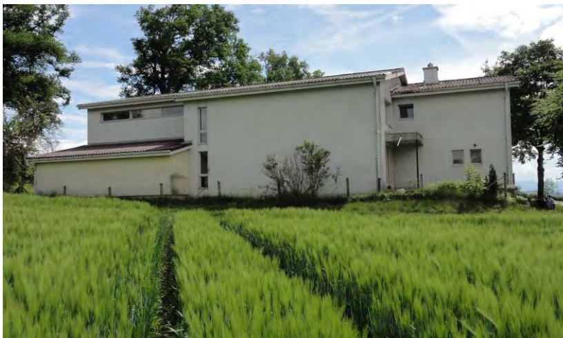
Figure 2: North view of the school building before renovation
