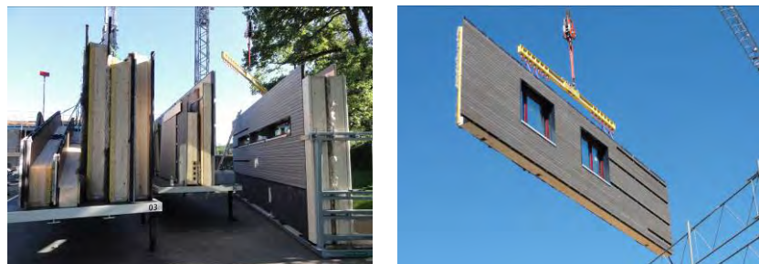
Figure 17-18: Module delivery on site
