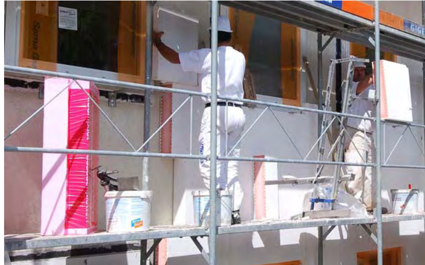
Figure 7: Insulation of façades with Hi-Compact insulation
