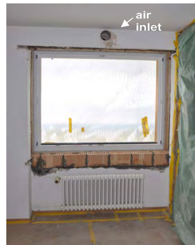
Figures 12-14: Ventilation main distribution with space saving rectangular ducts (top left), connecting the telescopic vertical round ducts between façade elements (bottom left), air inlet above window (right)
