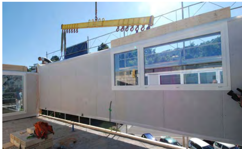
Figure 8: Mounting of the prefab structure
