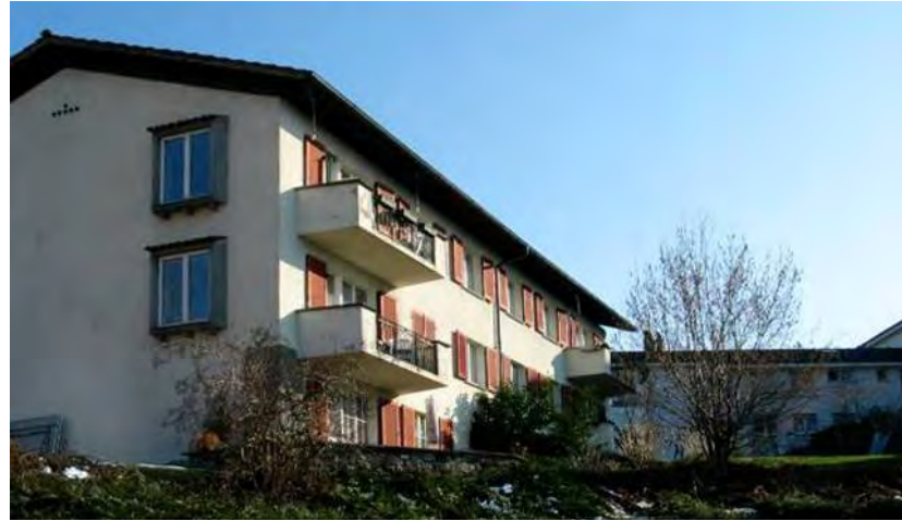
Figure 1: South-west view of apartment building before renovation
