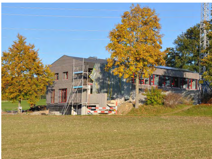
Figure 25: View of renovated building just before completion
