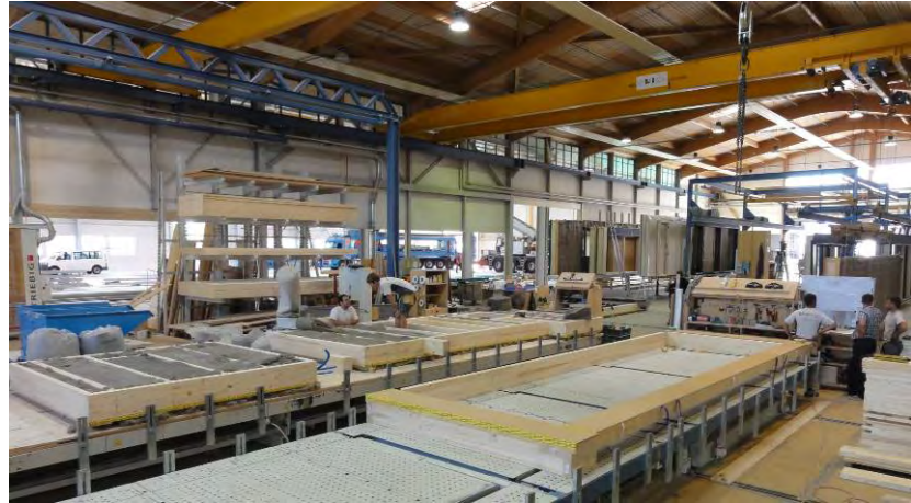
Figure 16: Prefabrication of modules in factory
