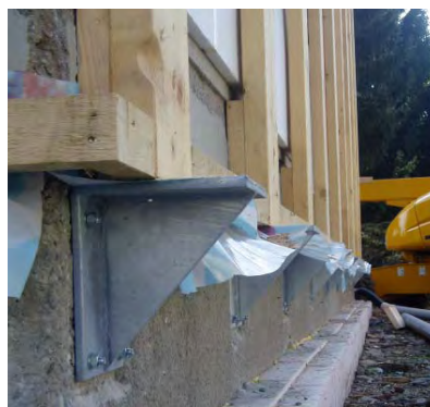
Figure 18: Steel-bearing angles on the plinth
