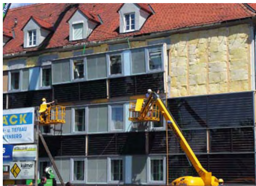
Figure 19: The solar collectors were integrated into the prefabricated modules. (Source: Gap-Solution GmbH)
