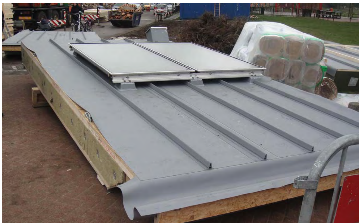
Figure 8: Prefab roof element with factory mounted solar thermal collector
