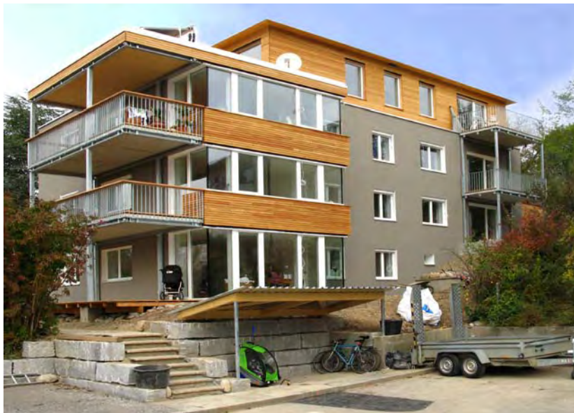
Figure 30: Renovated building from the south-eastern side. New are the large south oriented balconies, the living room extensions where the small balconies were before, the additional penthouse apartment and the additional balconies at the north-east corner.
