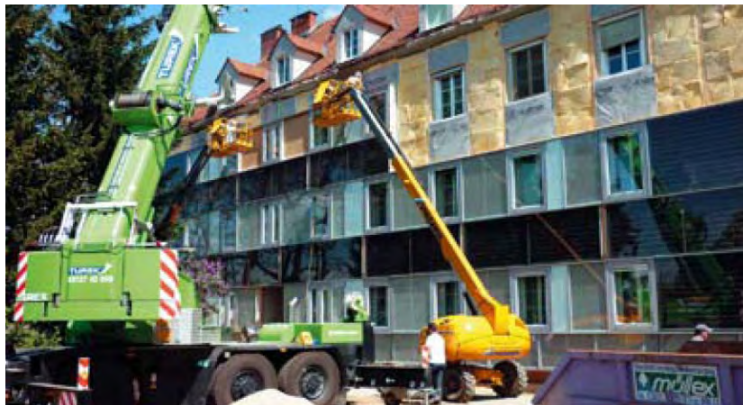
Figure 18: The on-site preparation is done by leveling laths. In-between the distribution system and supply pipes are installed.
