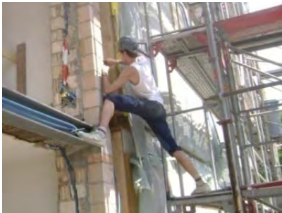
Figure 22: Preparation work for the living room extension
