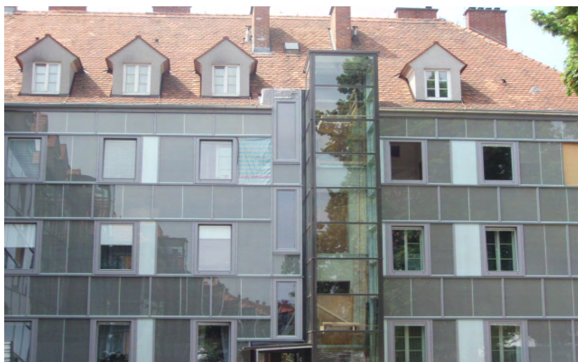
Figure 24: View of the renovated building from the back showing the additionally installed passenger lift
