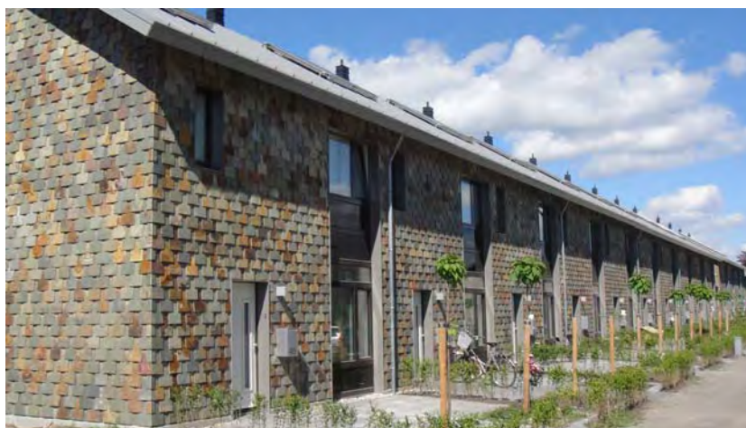
Figure 3: View of renovated building
