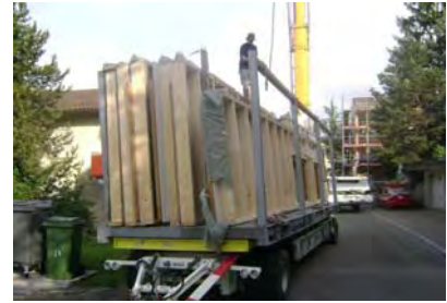
Figure 19: Transportation of large façade elements with flat bed trailer
