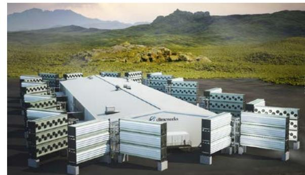
36.000 t CO<sub>2</sub>/Jahr DAC (Direct Air Capture)-Anlage von Climeworks (copyright: Climeworks, 2022)
