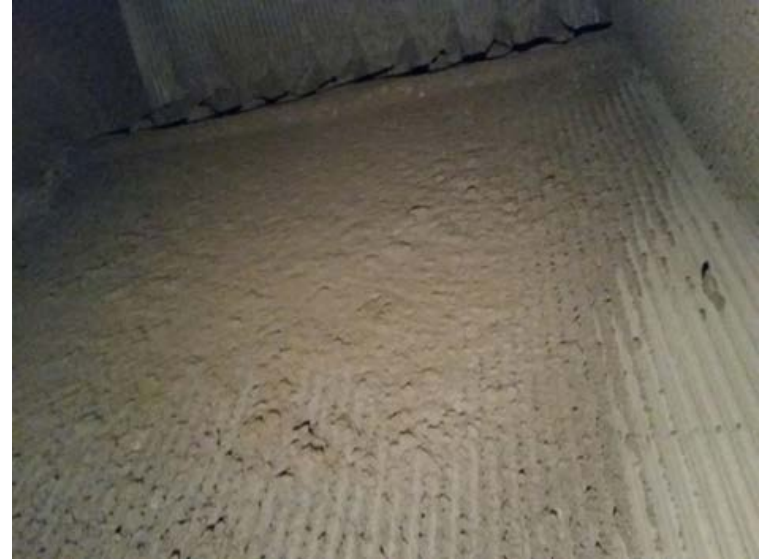
Rear wall of the 2 nd duct against the flow direction after a system operation of 9 weeks
