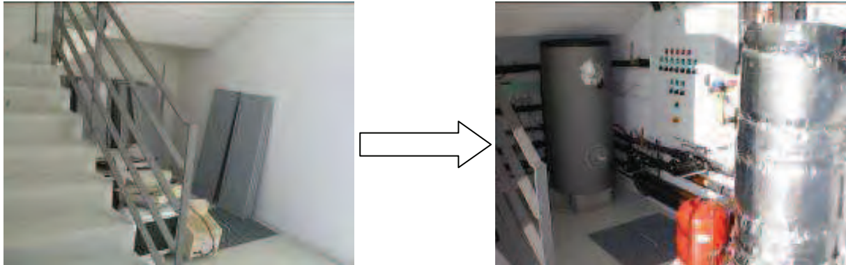
Technical premises before and after the works
