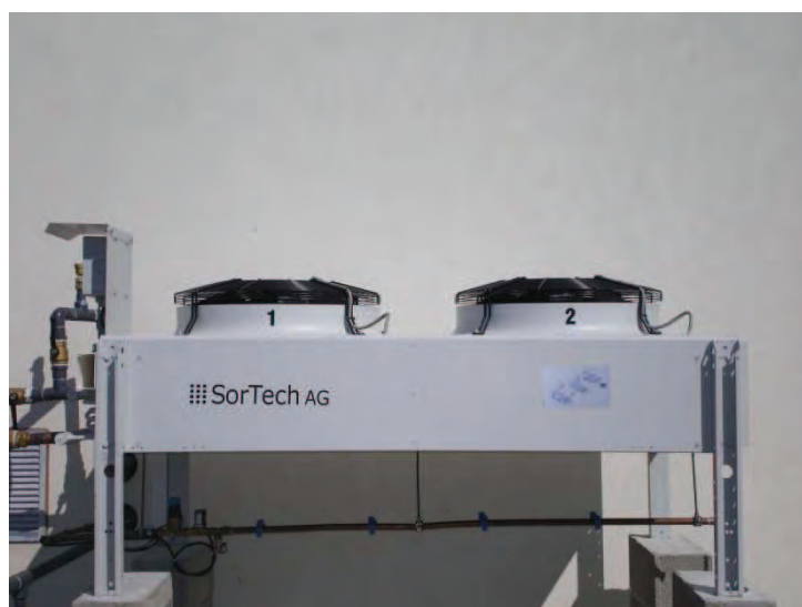
Drycooler used at the perpignan installation
