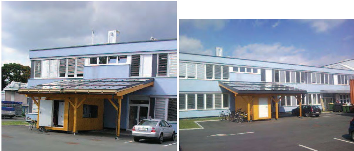
Figure 1: View of the CoolCabin in front of the office building [SOLID]
