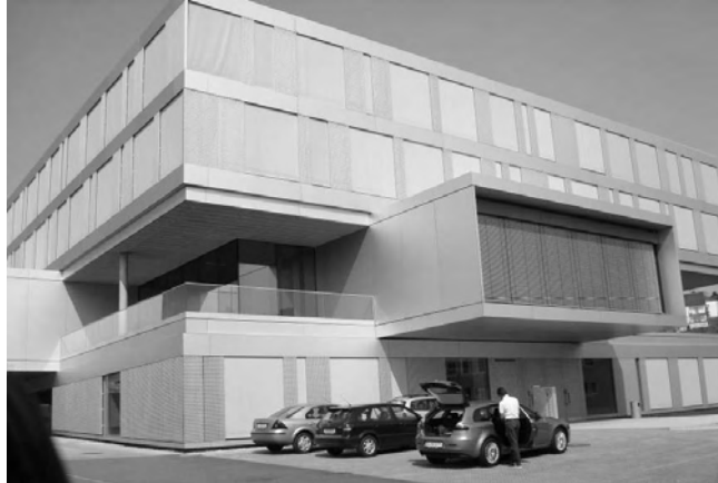
Figure 1: View of the office building
