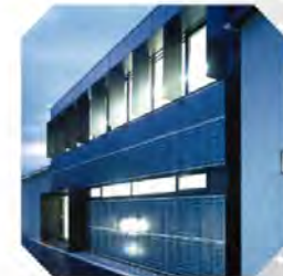
PHOTOVOLTAIK MADE IN AUSTRIA
