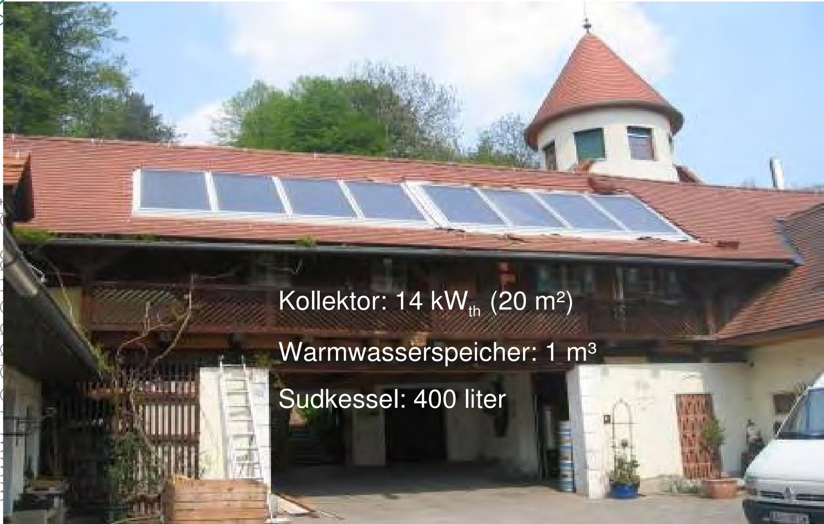
Kollektor:  $14 \text{ kW}_{\text{th}}$  ( $20 \text{ m}^2$ )
