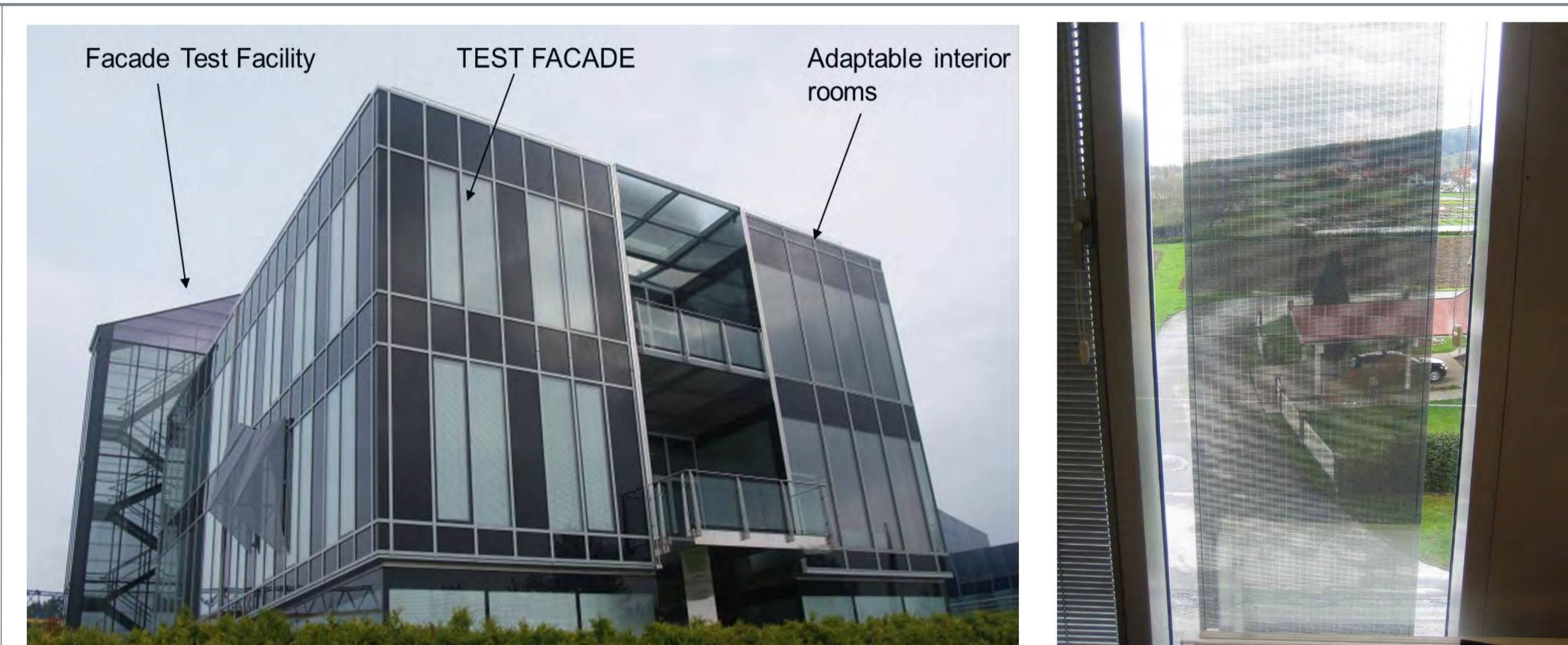
Fig. 1: Left: Test site in the FIBAG-Test building. The building combines a façade test facility, an adaptable test façade and adaptable interior rooms. Right: Semi transparent PV-module.
