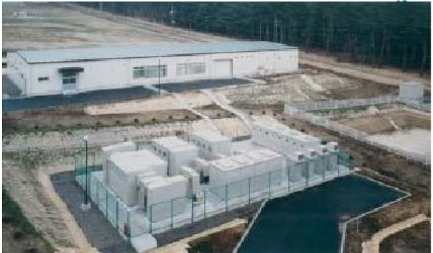
Research facility in Maebashi city
