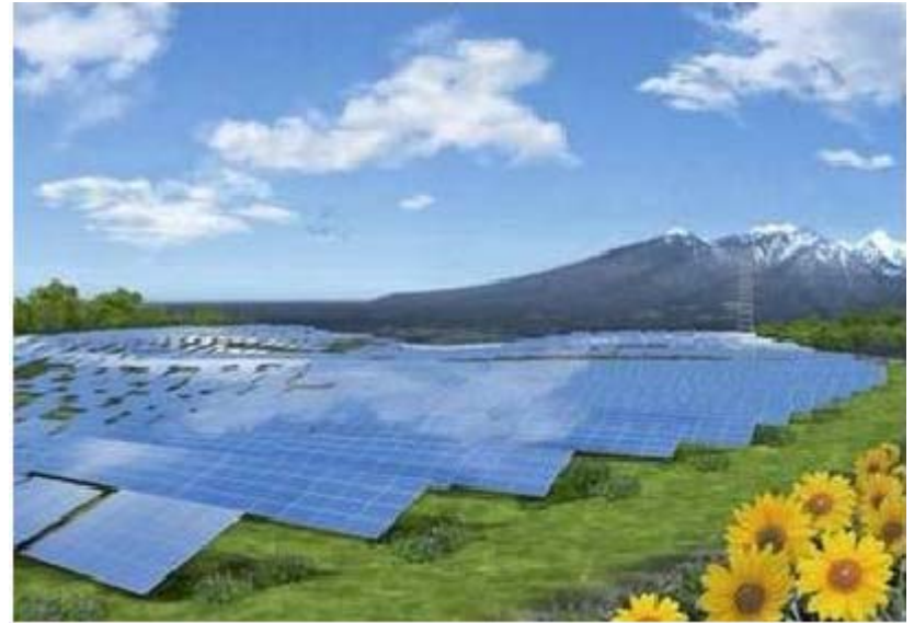
2009 November (PV ~2MW)
