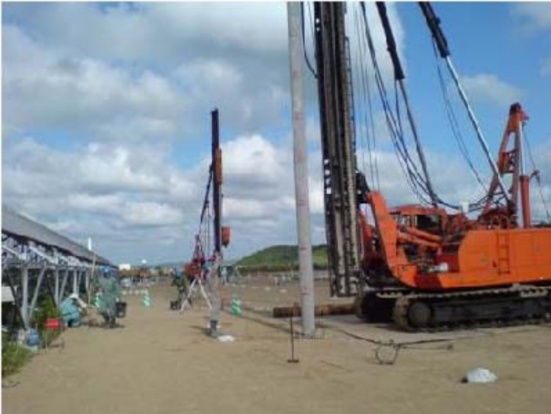
2007 July (PV: 80kW)
