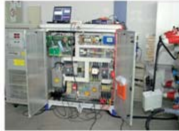
100 kVA photovoltaic inverter under test
