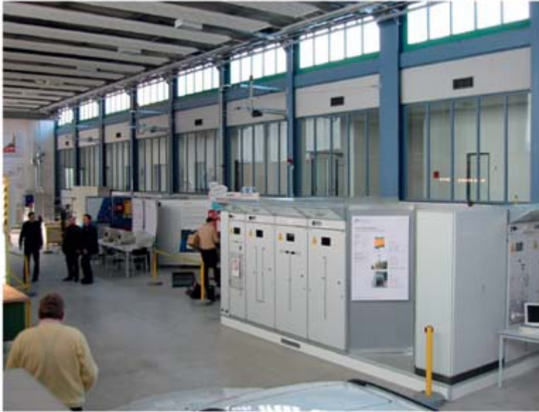
DeMoTec - Design Centre for Modular Supply Technology
