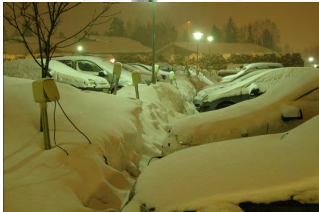
Fig. 19.3 Block heater poles typically have two-hour timers; the starting time is selected by the user, and the heating time is fixed for 2 hours from the start. Lock heater pole (left) and view from the car parking area of a row house condominium (right).
