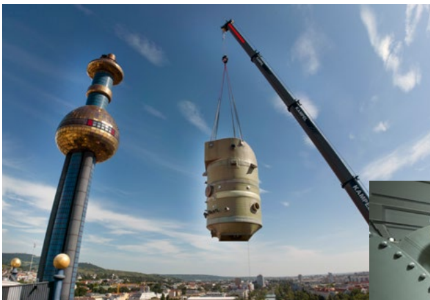
Construction of a large-scale heat pump at the Spittelau waste incineration plant in Vienna, photos: Wien Energie/Johannes Zinner
