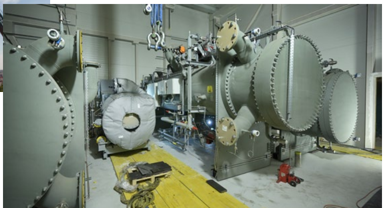
Construction of a large-scale heat pump at the Spittelau waste incineration plant in Vienna, photos: Wien Energie/Johannes Zinner
