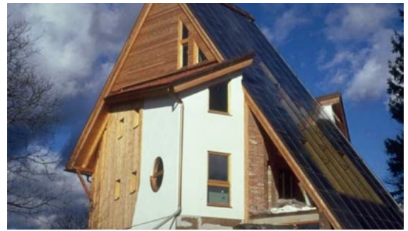
① Residential home heated 100% with solar energy (1997) – The Nader residence with 85 m 2 of collector area and 75 m 3 of energy storage systems is heated 100% by solar energy and was one of Austria's contributions to IEA SHC Task 26 Solar Combinations. (Photo: AEE INTEC)
