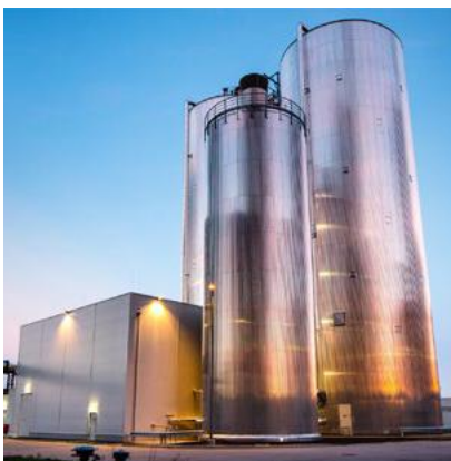
High-pressure heat storage facility, district heating Vienna, Photo: Wien Energie/Ian Ehm
