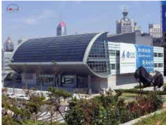
Solar System for Cooling Olympic Games 2008 China / Qingdao: S.O.L.I.D
