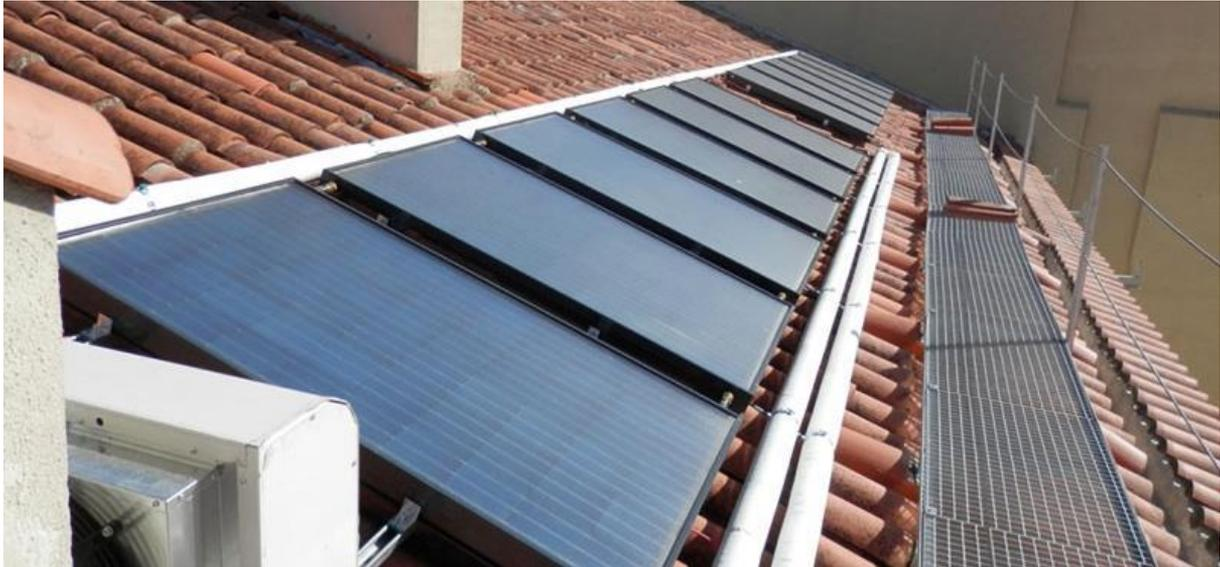
Abbildung 6: View of the roof-mounting PVT installation in the urban centre of Zaragoza (Source: EndeF).
