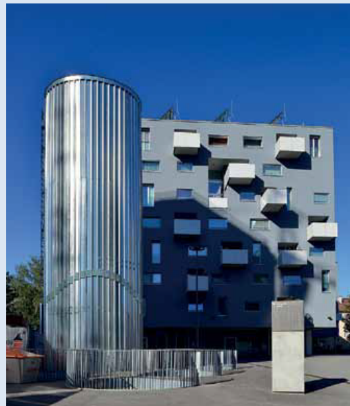
Figure 3: 200 \text{ m}^3 energy storage tank (source: www.stadtwerklehen.at )
