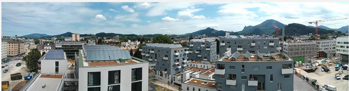
Figure 1: Aerial view on Northern part of the urban quarter “Stadtwerk Lehen”. In sum, 2,048 m 2 solar thermal collectors are split into 13 roof-mounted collector fields (Source: AEE INTEC)
