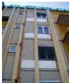
Picture 23: Heat dissipation system installed on the outside of the exterior wall (Source: AEE INTEC)
