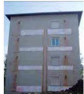
Picture 6: Two views on the exterior walls during installation works. The heat dissipation (XPS-boards with inserted heating pipes) are assembled in the wall-areas below the windows (Source: AEE INTEC)
