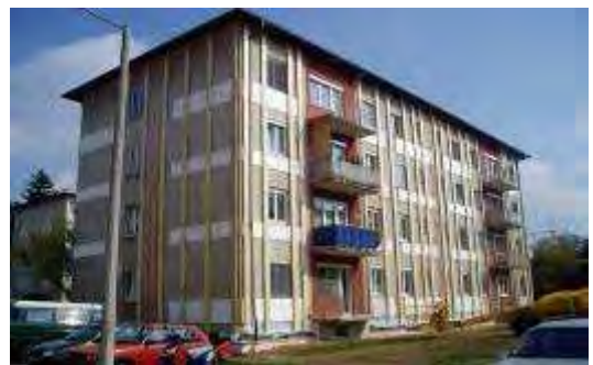
Picture 23: Heat dissipation system installed on the outside of the exterior wall (Source: AEE INTEC)
