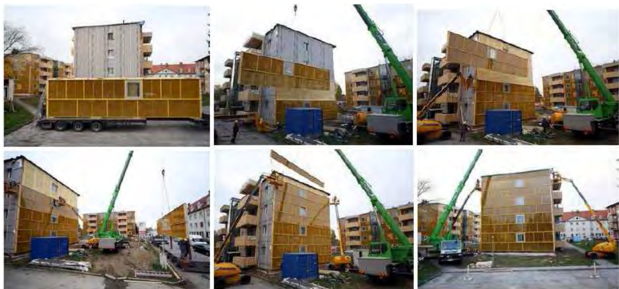
Picture 17: Transport on-site and assembling procedure (Source: gap-solution GmbH)
