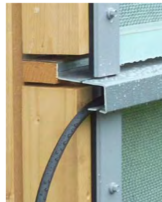
Picture 11: The upper picture shows the vertical joints with the cover strips fixed by screws. The picture below shows the horizontally mounted façade plate to ensure the sealing against driving rain
