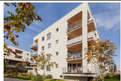
AT5: Energy City Graz, new residential building
