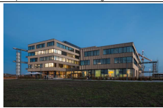
AT1: Aspern IQ, new office building
